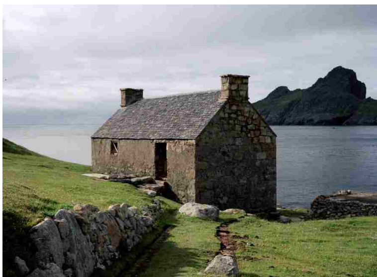
Figure 52 The storehouse on St Kilda was constructed in the 1780s as part of wider efforts to promote a fishing industry. SC1463846
